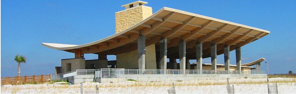
State Park Beach Pavilion - Orange Beach, AL
