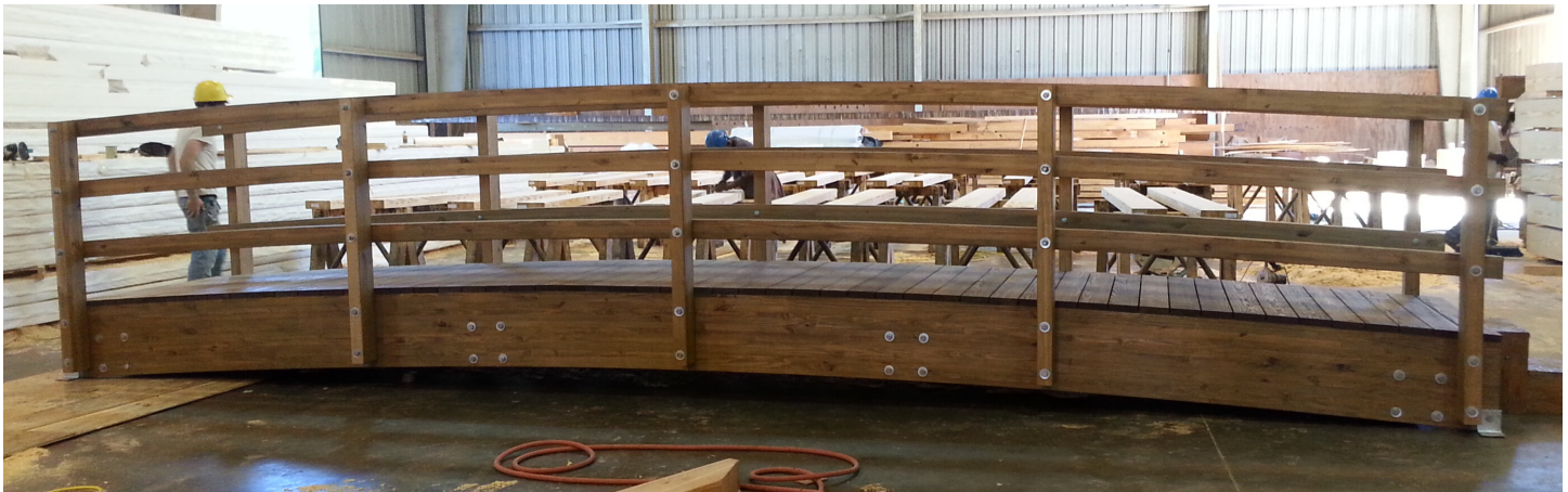
Assembly of Pedestrian Bridge with horizontal rails going to Magnolia, AR
