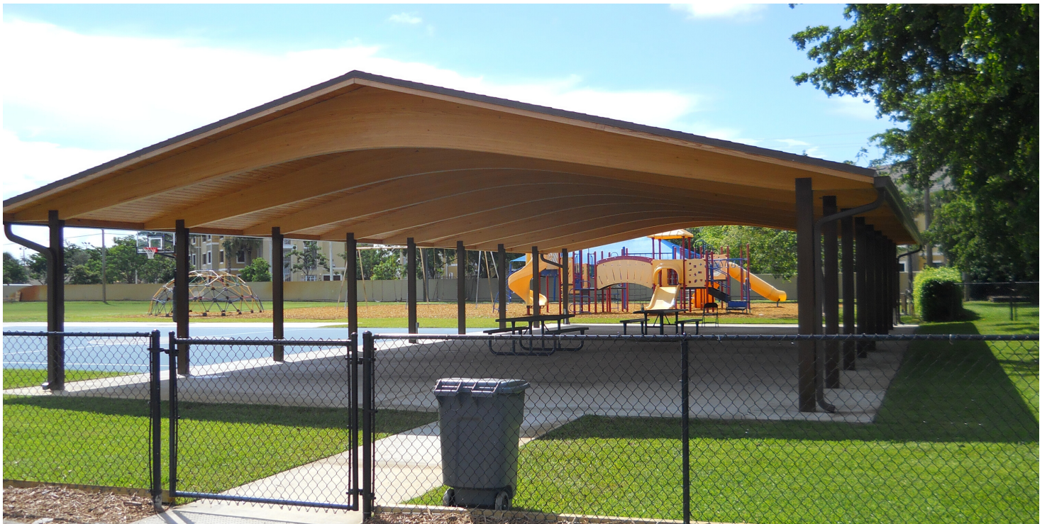
Pitched & Curved Shelter with Steel Columns
