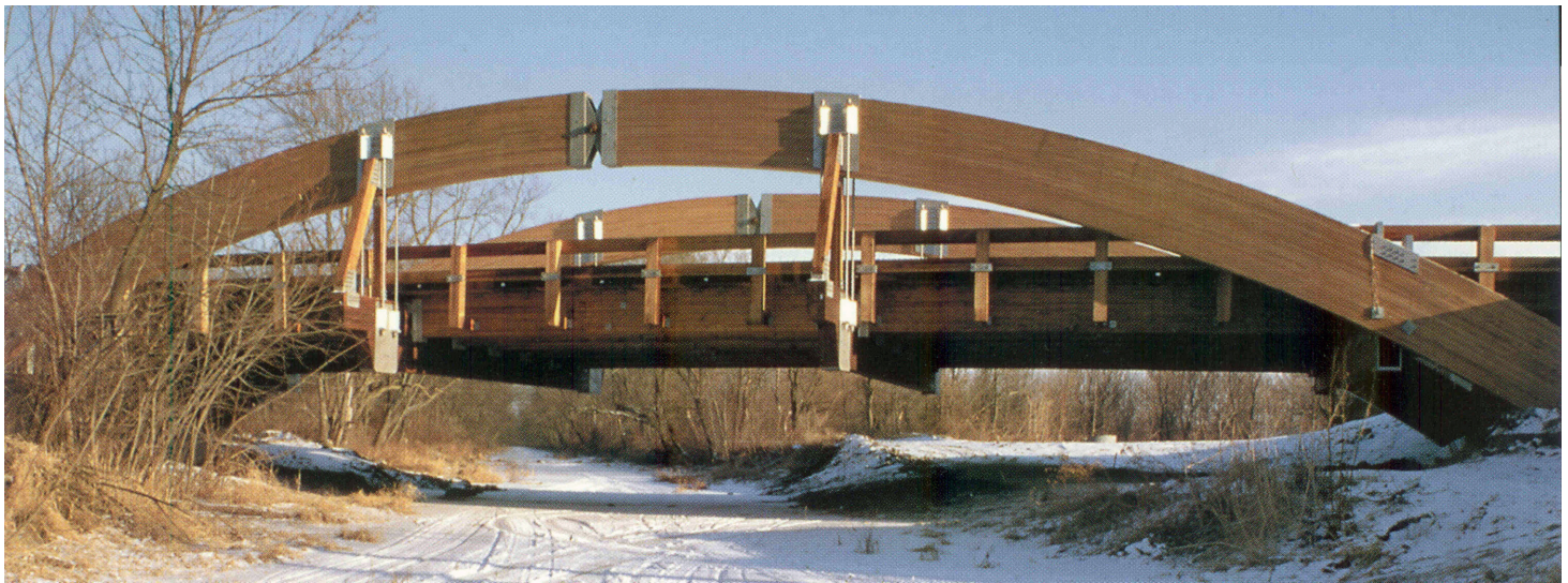
Five Mile Bridge - Grundy County, IL
