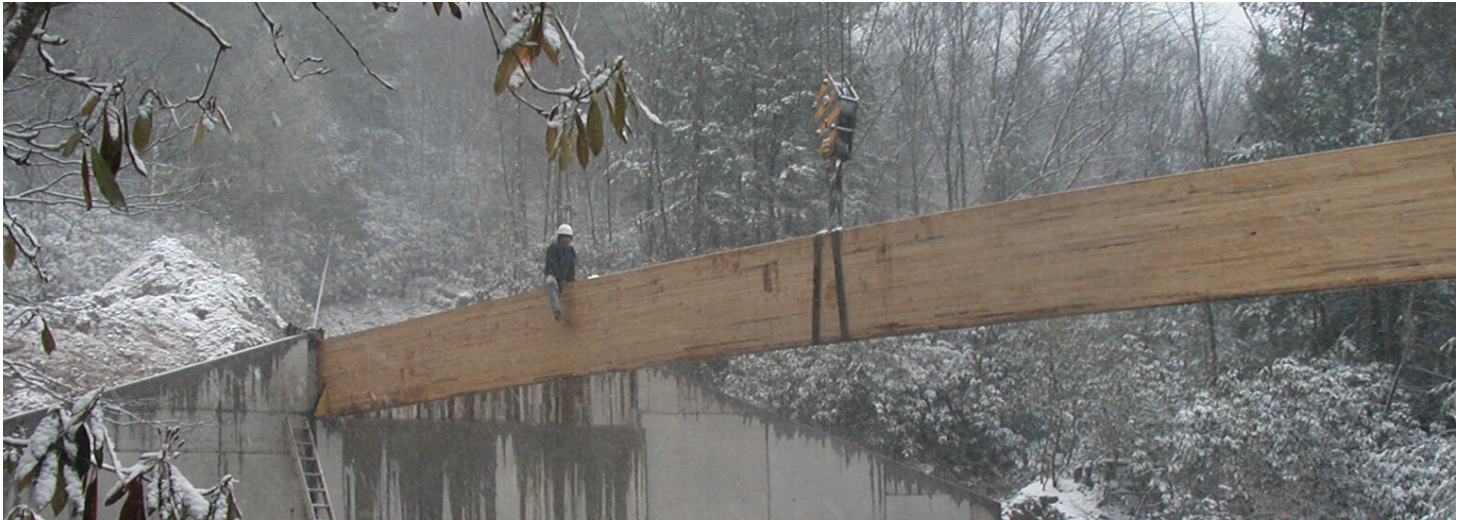
Laminated Wood Girder for Vehicular Bridge
